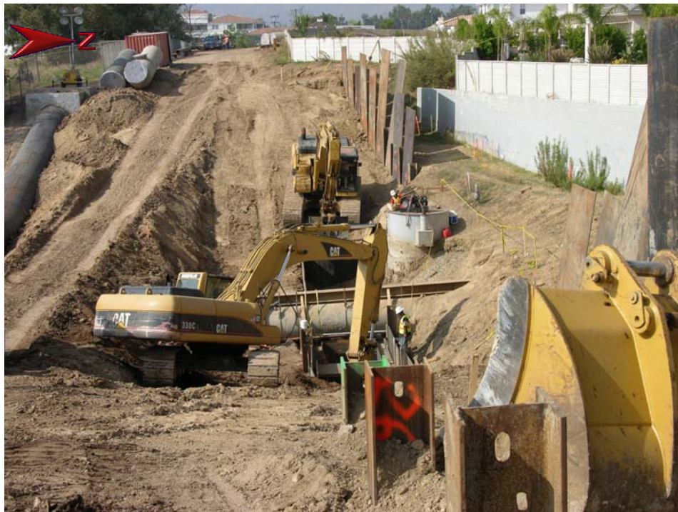
Figure 4: Excavation for relocated portion of the West Valley Feeder No. 1
