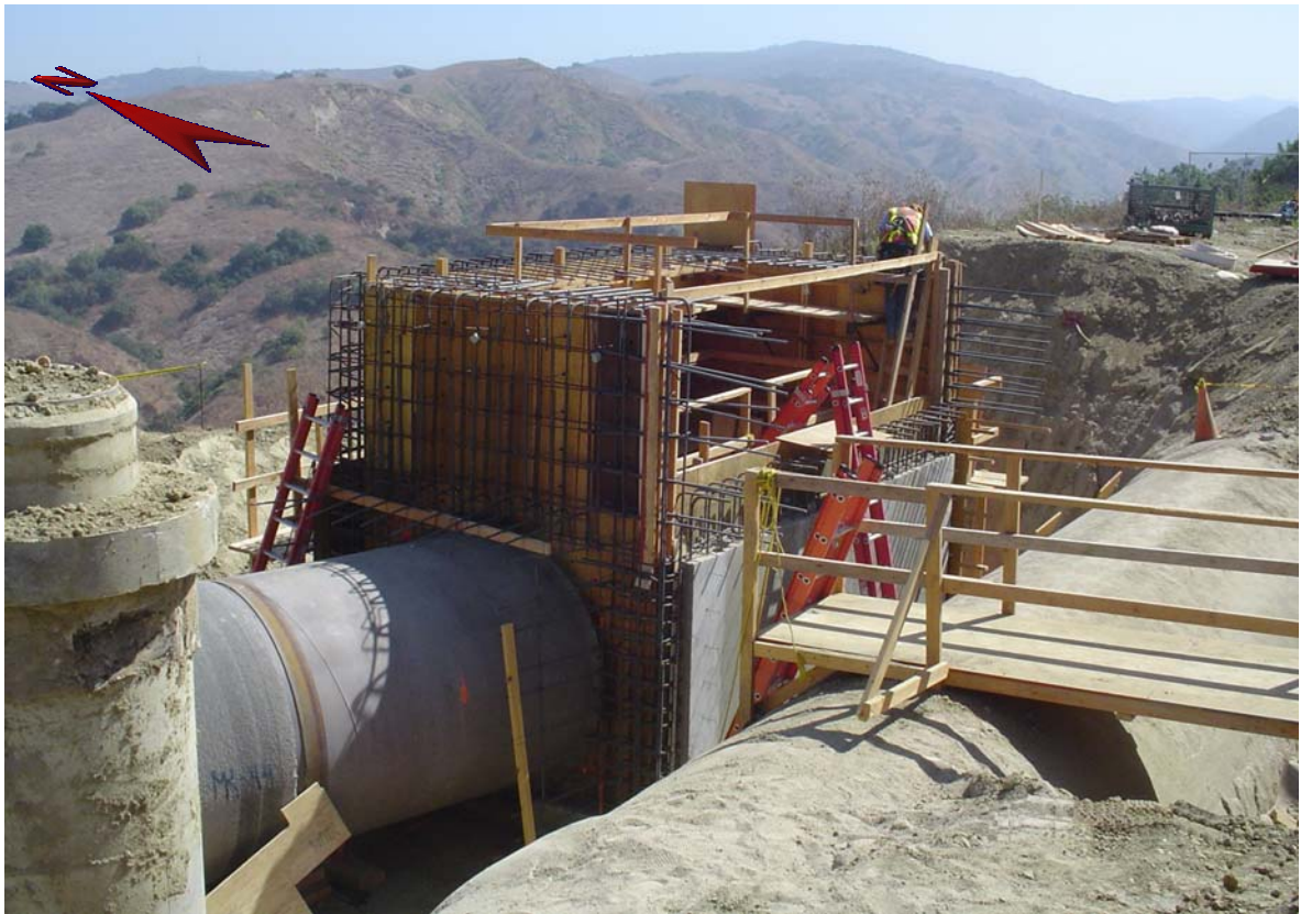
Figure 7: Construction of the overflow structure in progress
