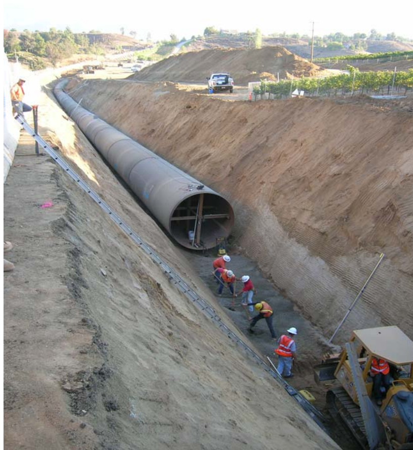
Figure 1: Pipeline installation continues
