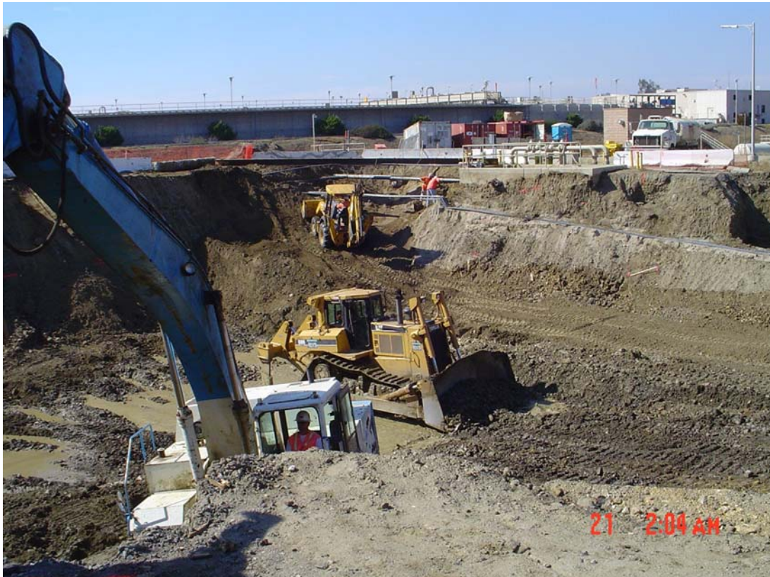
Figure 8: Coal removal structure excavation underway at the Skinner ORP
