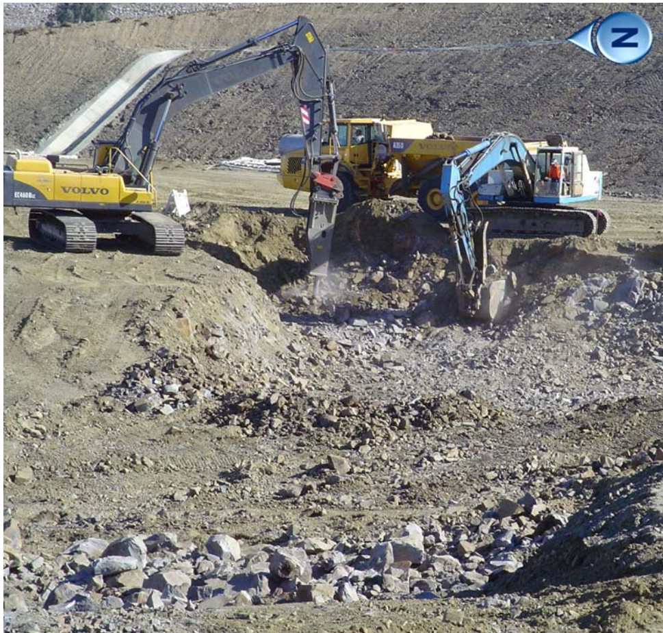
Figure 2: Washwater Reclamation Plant No. 3 construction site excavation
