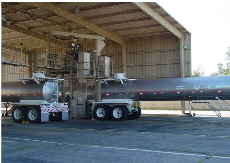
Figure 9: Two of the chlorine cargo trailers at the Chlorine Unloading Facility
