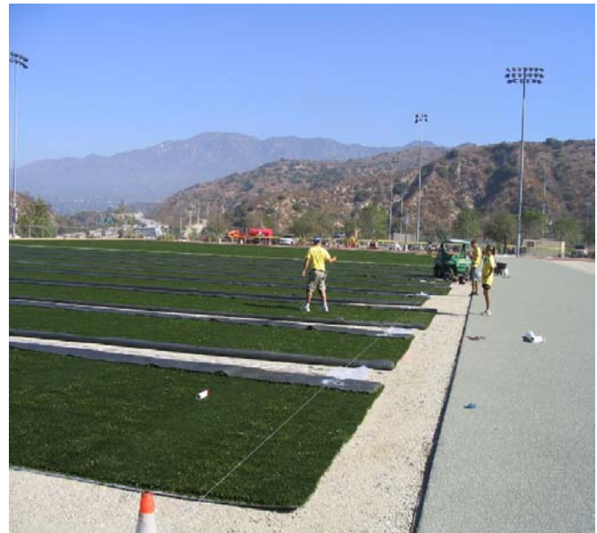
Synthetic Turf Installation in Sports Complex Soccer Fields (City of Glendale)
