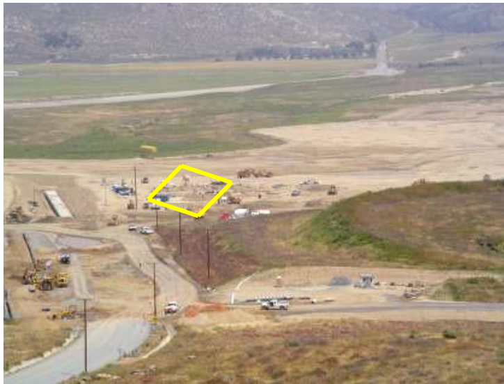
Figure 1: Valley-Wide site grading – Milestone No. 1 – Looking Northwest
