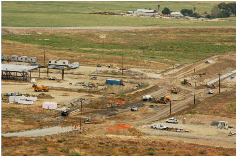
Figure 2: Searl Parkway Phase I Searl Parkway Construction – Looking Northeast
