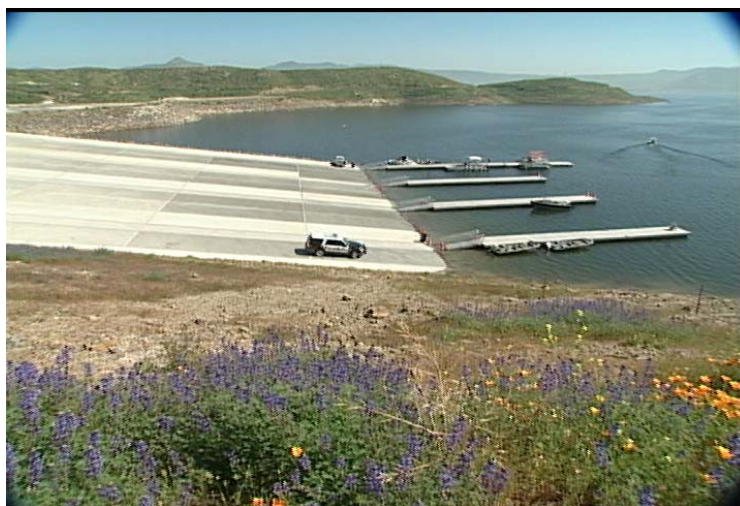
Figure 2: Floating docks and marina ramp – Looking Northeast
