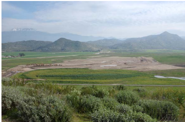
Figure 1: Valley-Wide site grading – Looking Northwest
