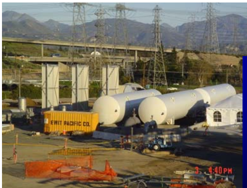
Construction of ORP facilities at Jensen Treatment Plant
