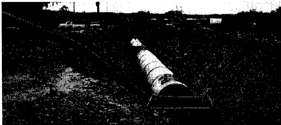
Pipe installation in Site 2 of Mentone - RUSD pipeline
